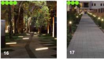
1. Embedded sidewalk lighting 2. Light the extents of a path or zone
