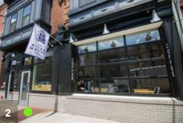
2 Ground floor facade with stem wall and mixed transparency and opaque surfaces
