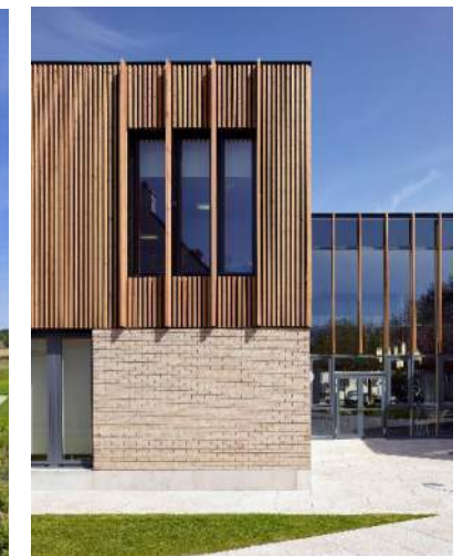
Transparent building entry framed by brick massing
