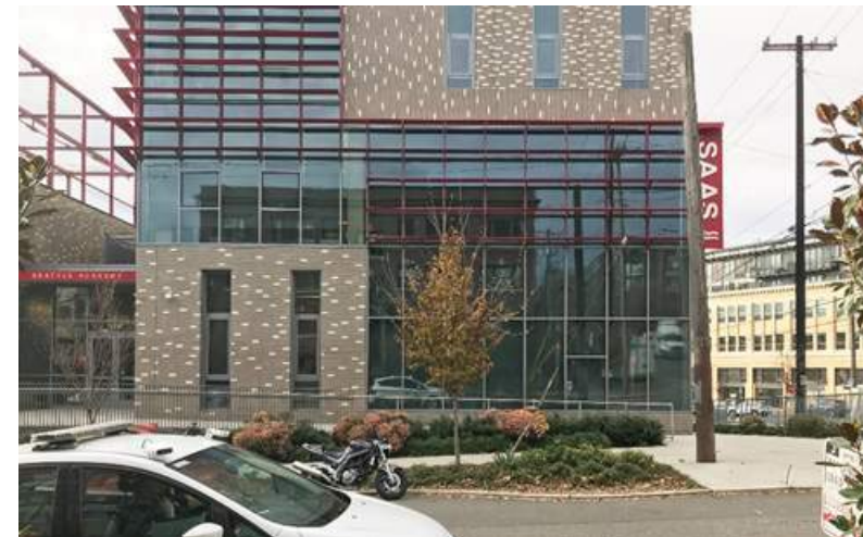
Gray and white brick create a visual texture, glass with red sunshades span the facade to break-up the massing
