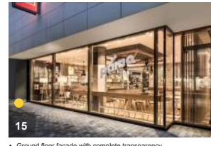
15 • Ground floor facade with complete transparency
