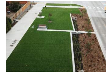
Stormwater mitigation facilities (right) with green space for play (left)
