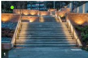
1 • Handrail-mounted lighting at exterior staircases
