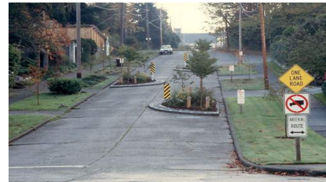
Chicanes can help slow and calm vehicle traffic to create safer streets for pedestrians
