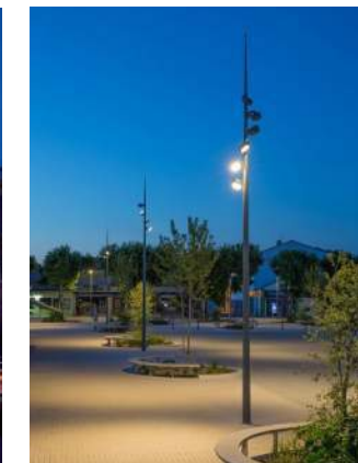
Tall fixtures effectively illuminate a large area
