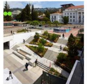
1. Introduce stairs and/or ramps to navigate elevation changes 2. Integrate stairs and ramp landings to maximize space efficiency 3. Use negative space for planting beds, site furniture
