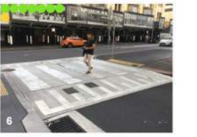
1. Highlight crossing areas with contrasting paving 2. Use raised crosswalks for added pedestrian safety
