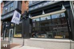
11 • Ground floor facade with stem wall and mixed transparency and opaque surfaces
