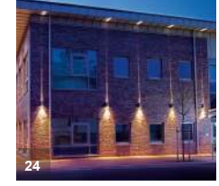
24 • Downlighting to light facade and sidewalk
