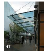
17 • Glass awning - allows light to pass thru; but dirt visible from below
