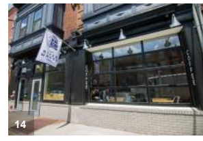
14 • Ground floor facade with stem wall and mixed transparency and opaque surfaces
