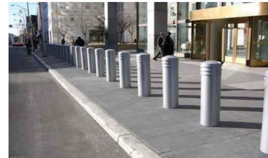
Bollards located at busy sidewalks, intersections, and building entrances provide additional protection for pedestrians
