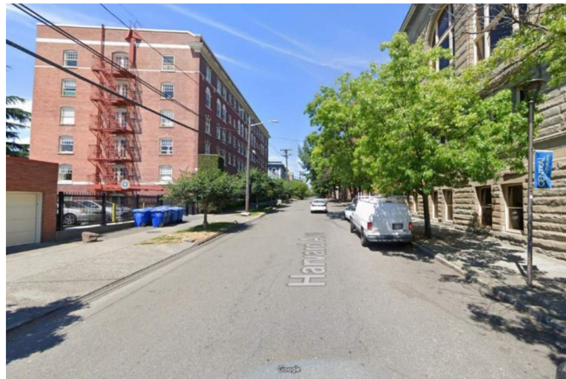
Existing condition on Harvard Avenue near the intersection with E Pine Street
