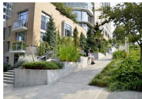
Street-level facade and entries step with the street slope
