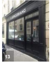
13 • Commercial entrance not setback from sidewalk
