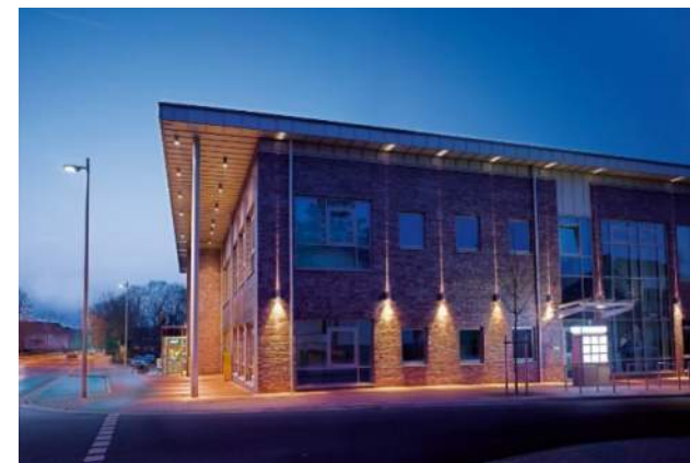
Building-mounted lighting brightens the sidewalk
