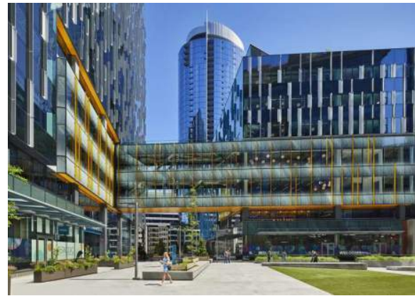
Transparent skybridge offers visual connections in and out of building
