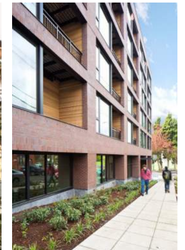
Red-brown brick with wood accents above ground level - wood accents reduce the visual weight of the brick
