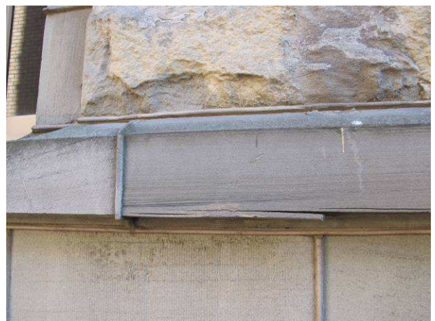
Delaminating stone on north façade
