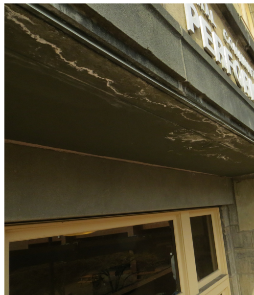
Fig. 9 Efflorescence on the underside of the east entry cornice
