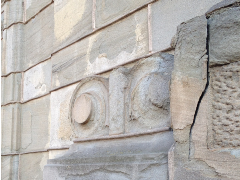
Fig. 5 Cracked Stone Frieze Above North Elevation Window Mantel
