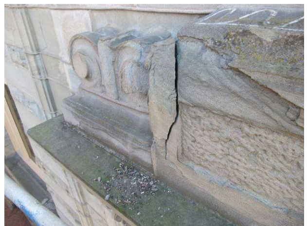
Damaged spalling stone, north façade
