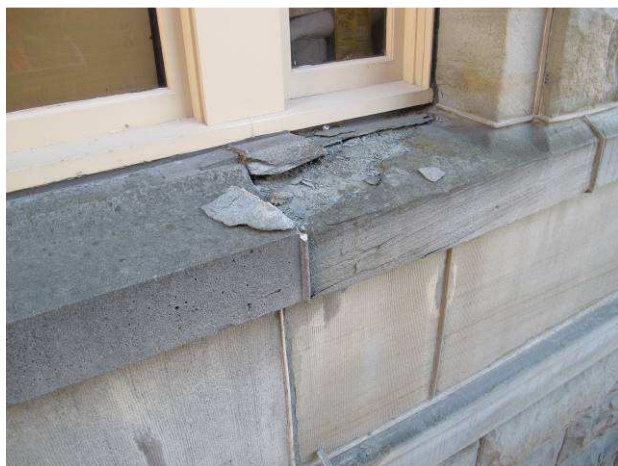
Damaged window ledge, north façade
