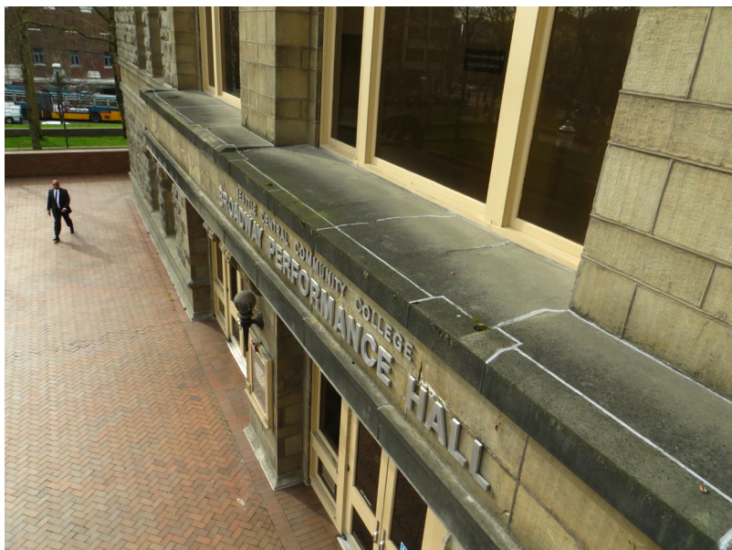
Fig. 8 Sealant joints over the east entry cornice
