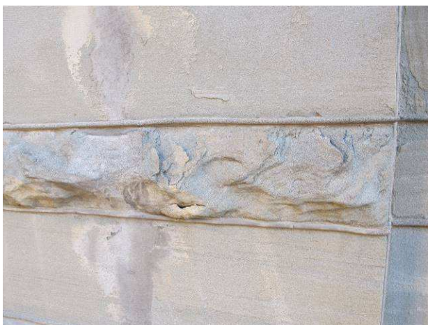
Spalling stone, north façade
