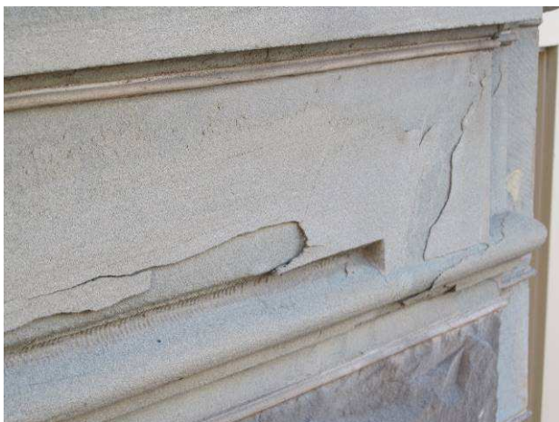
Spalling stone, north façade
