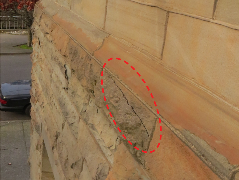
Fig. 1 Cracked Stone Over South Entrance (circled in red)
