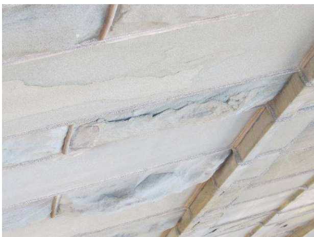
Spalling stone, west end, north façade
