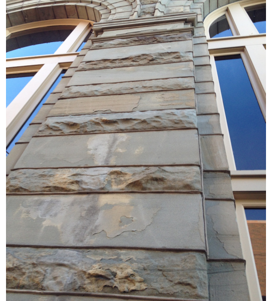
Fig. 6 Water unable to weep through mortar joints damages the stone surface
