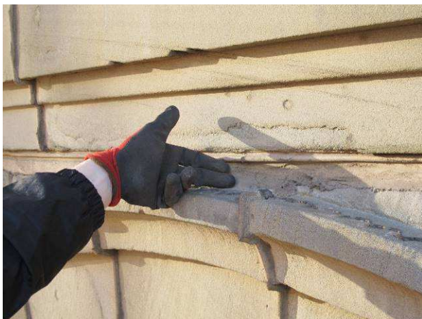
Damaged stone and overly large mortar joint
