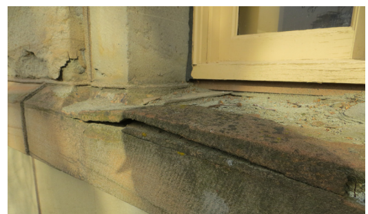
Fig. 4 Spalled Window Sill at North Elevation
