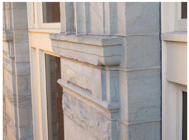
Damaged, spalling stone on north façade
