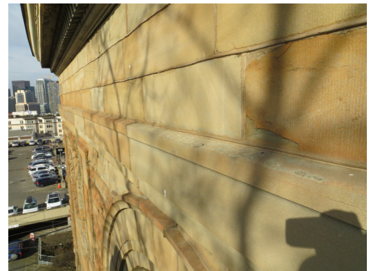
Fig. 7 Water unable to weep through mortar joints damages the stone surface
