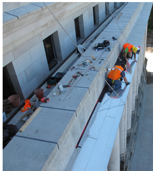
Fig. 10 Example of a metal cover installed over a wide stone ledge at Washington State Legislative Building in Olympia, WA
