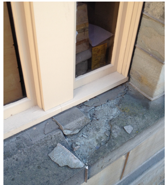
Fig. 3 Spalled Window Sill at North Elevation
