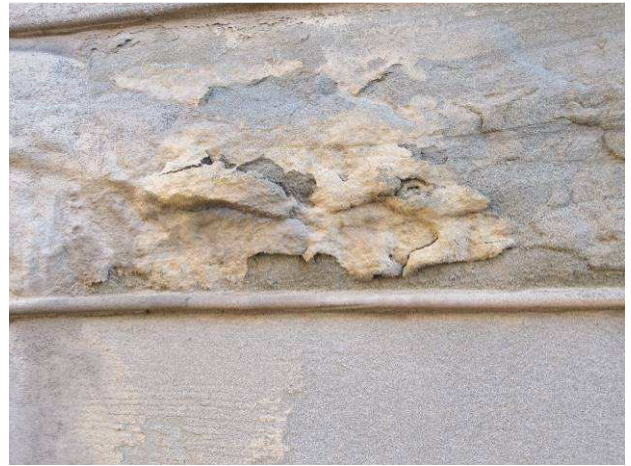
Spalling stone, north façade
