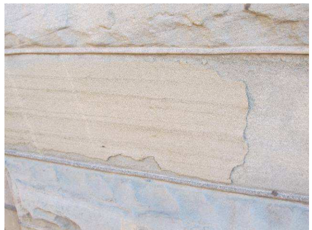
Spalling stone, north façade
