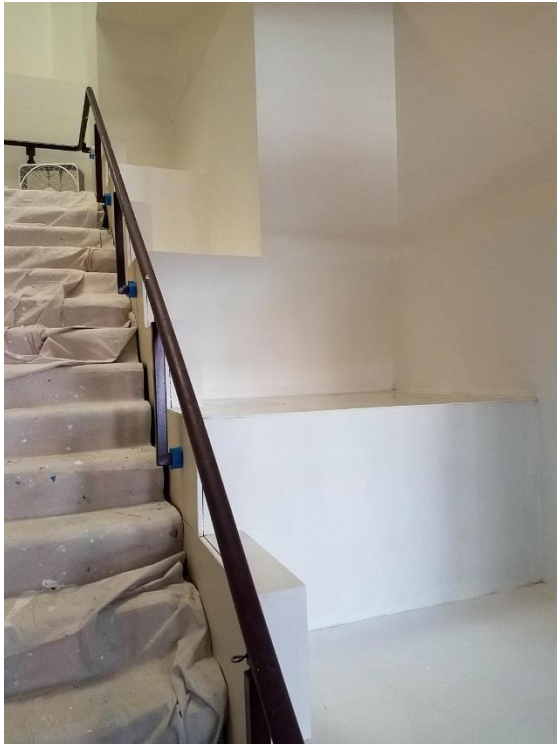
Picture 1: Staircase at Siegel; Location of work.
