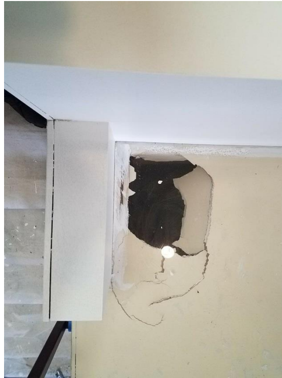
Picture 2: Damage; drop is ~6ft through.
